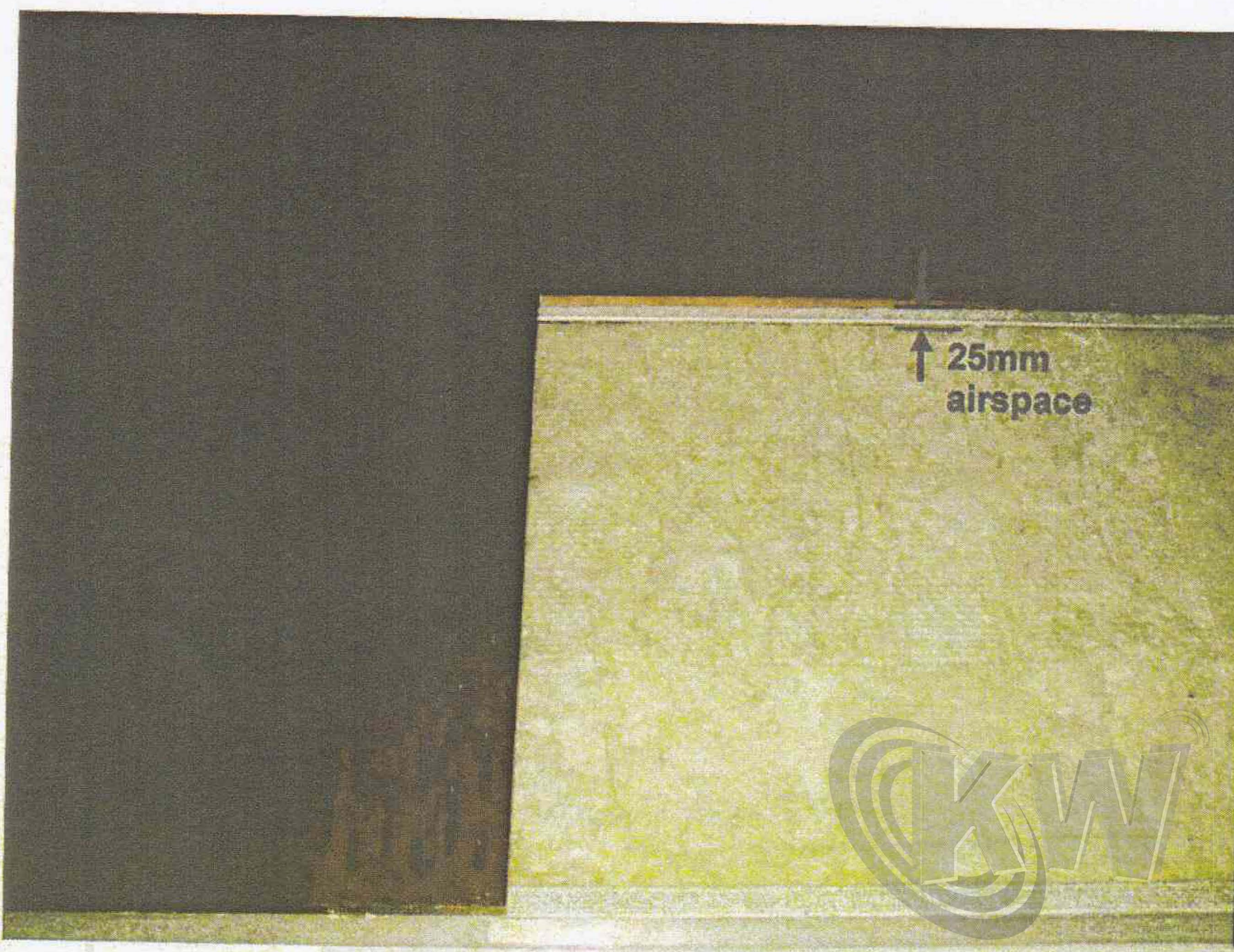
Figure 5 : Slotted "Murano/SIU akustik" HDF panel laying on steel channel leaving 25mm airspace between the rockwool and the panel
