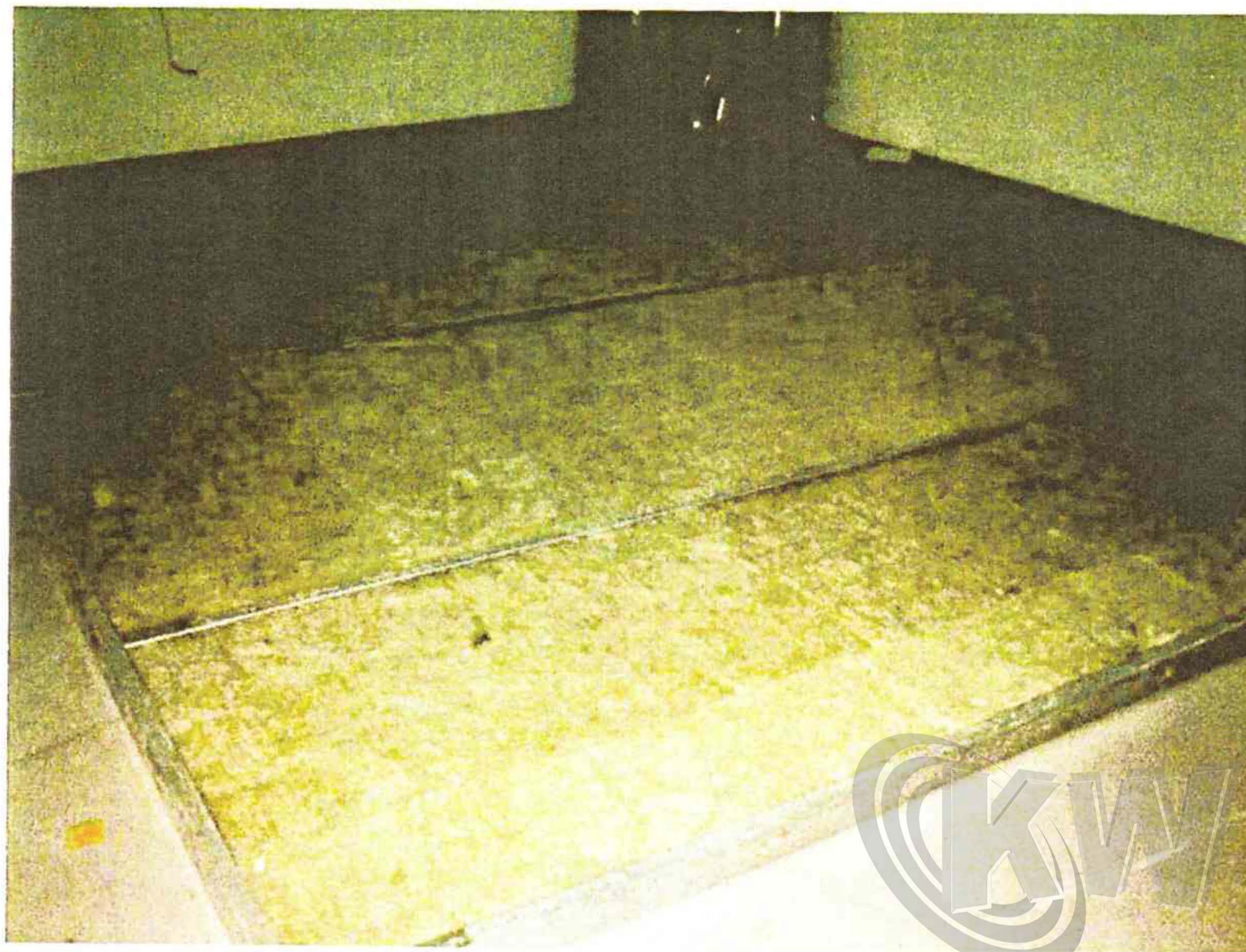
Figure 4 : 50mm (thick), 60kg/m 3 density rockwool were installed inside 75mm thick steel channel frame
